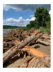
At the upstream portion of the project where the stress on the bank is highest, they will put in root wads to support the bank while the vegetation is establishing.
